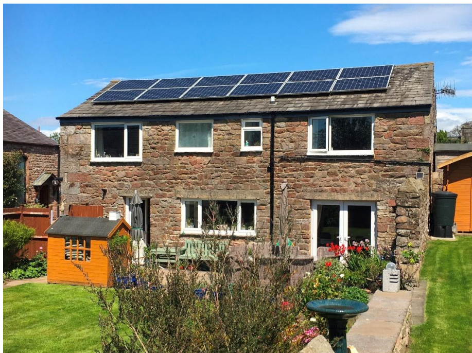
Solar panels on a house in Aldcliffe
